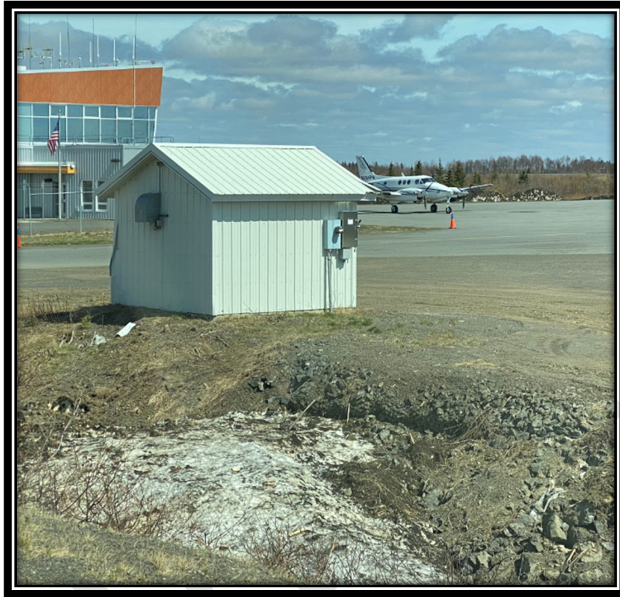
Figure 3: Sewer Pump Station
