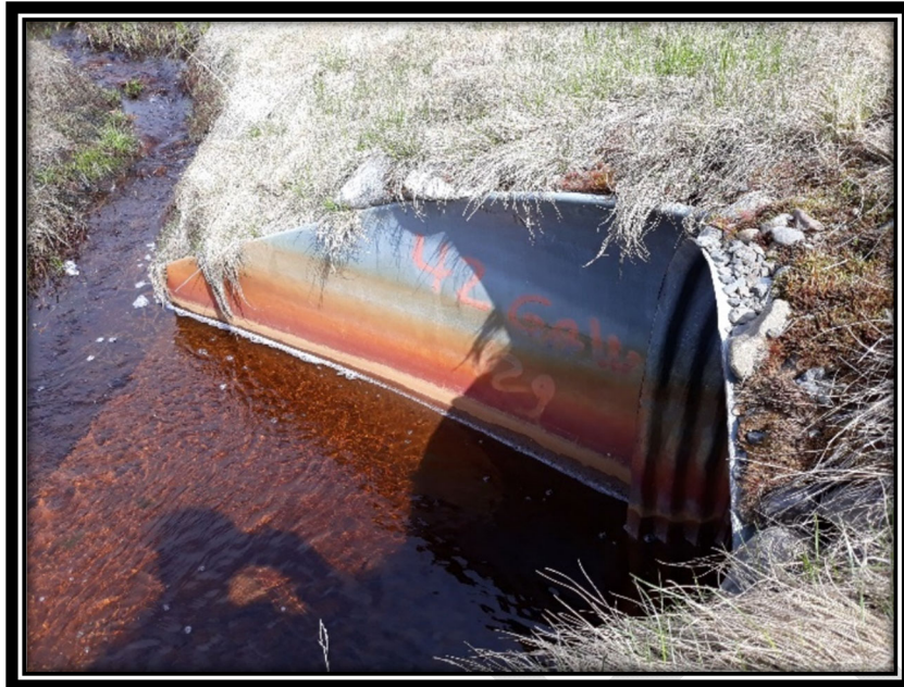
Figure 6: Runway Culvert Inlet West of RW 1-19
