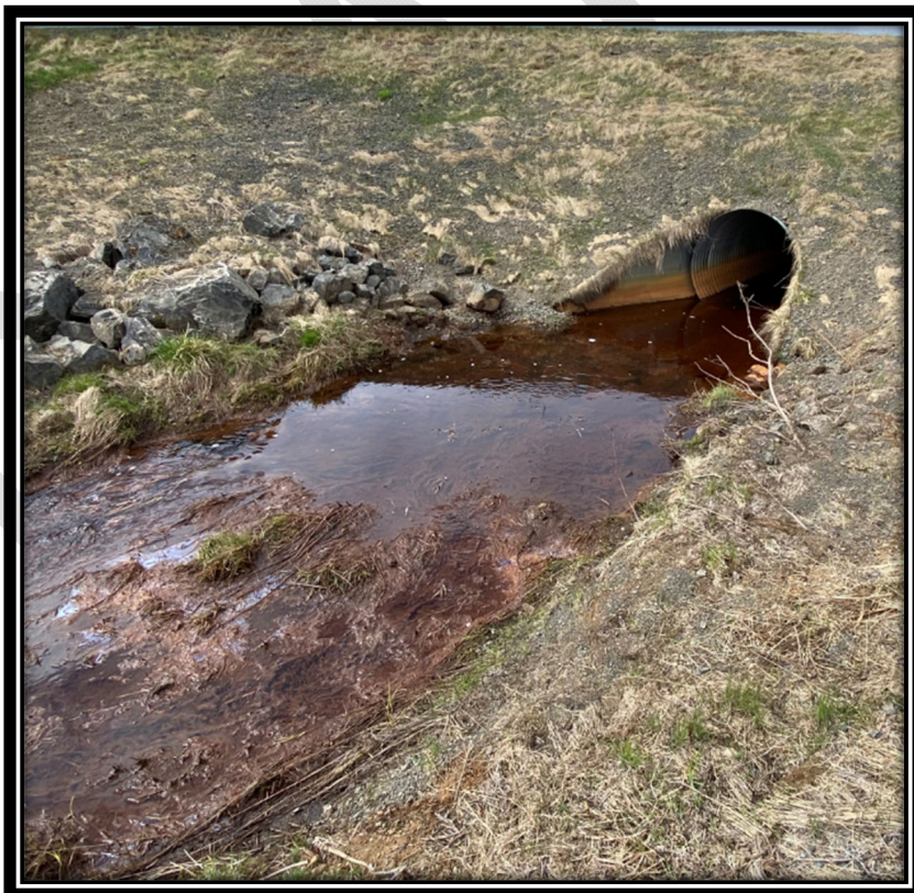
Figure 7: Runway Culvert Outlet East of RW 1-19
