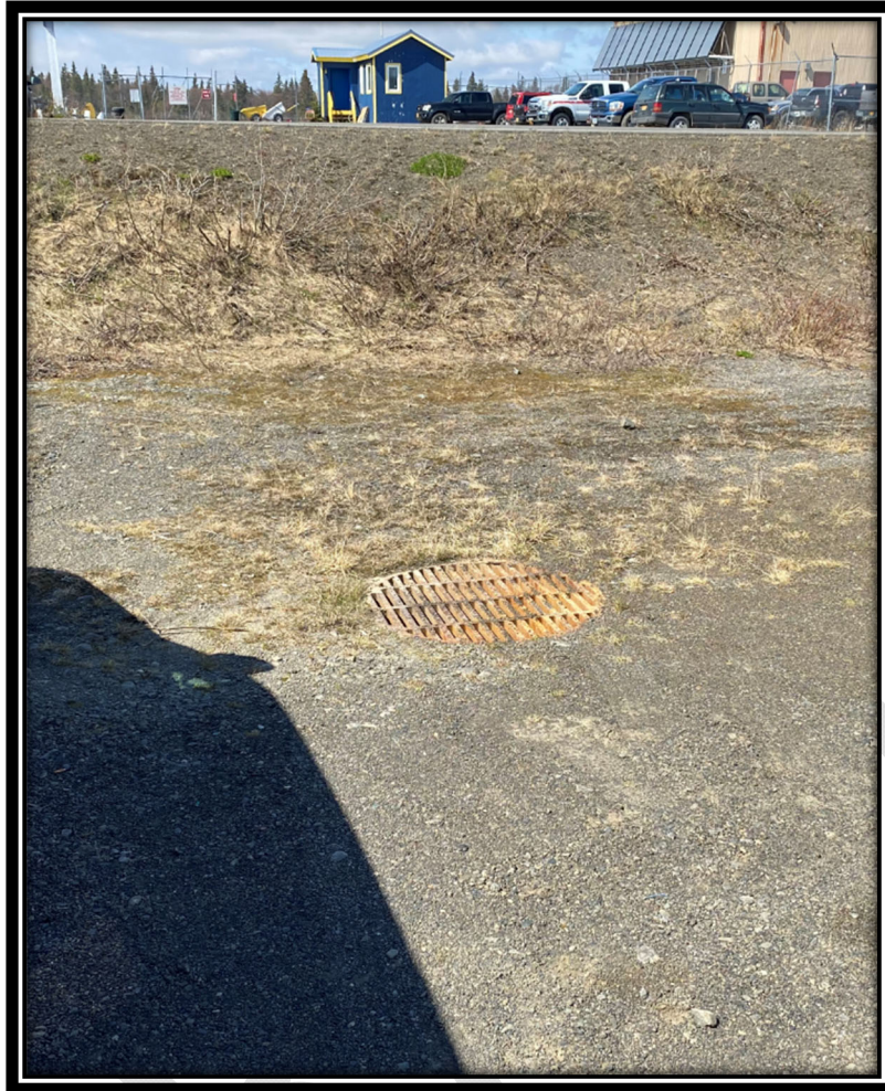
Figure 5: Storm Drain Catch Basin
