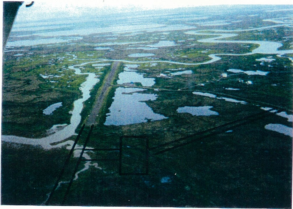
Figure 3. Proposed runway extension, parking apron (approximate), and access road at Kwigillingok, Alaska.
