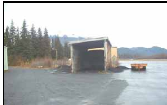
Figure 16: Sand Storage Building
