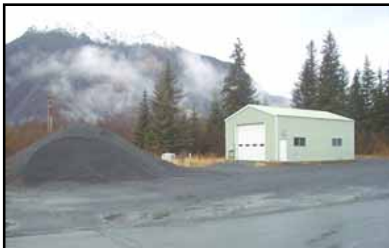
Figure 15: DOT&PF Maintenance Building
