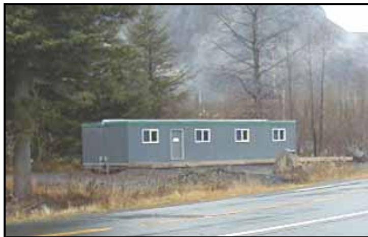
Figure 19: GGDST Office on Alaska Railroad Property
