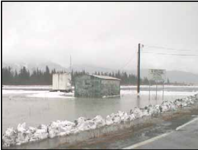
Figure 6: Flooded Lighting Building
