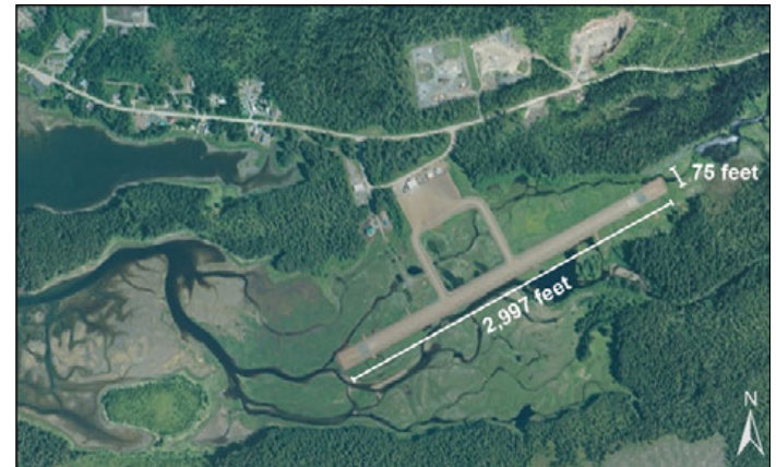
Figure PN1. The airport at Hoonah, Alaska, a primarily Alaska Native village about 50 miles northwest of Angoon.
