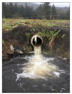
Figure 3.—Perched culvert on the stream at WP 4104.
