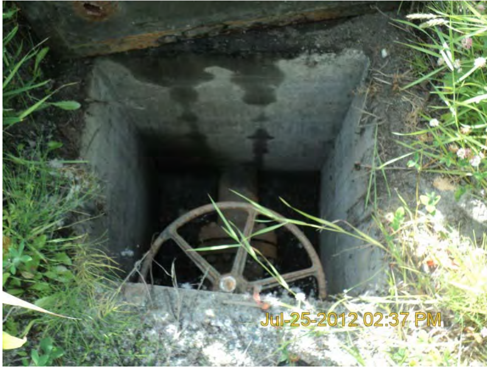
PMP 25.5 – View Inside Gate Valve 4
