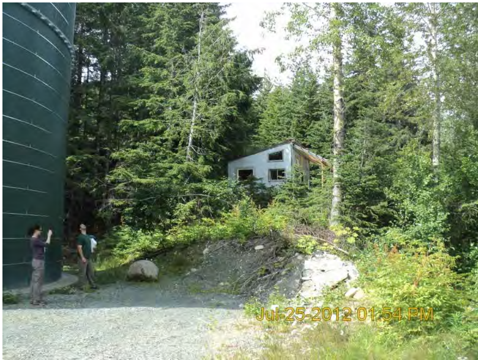
PMP 1.9 (Young Road Site) –Water Tank and Adjacent Soil Berm with Remaining Soil Contamination
