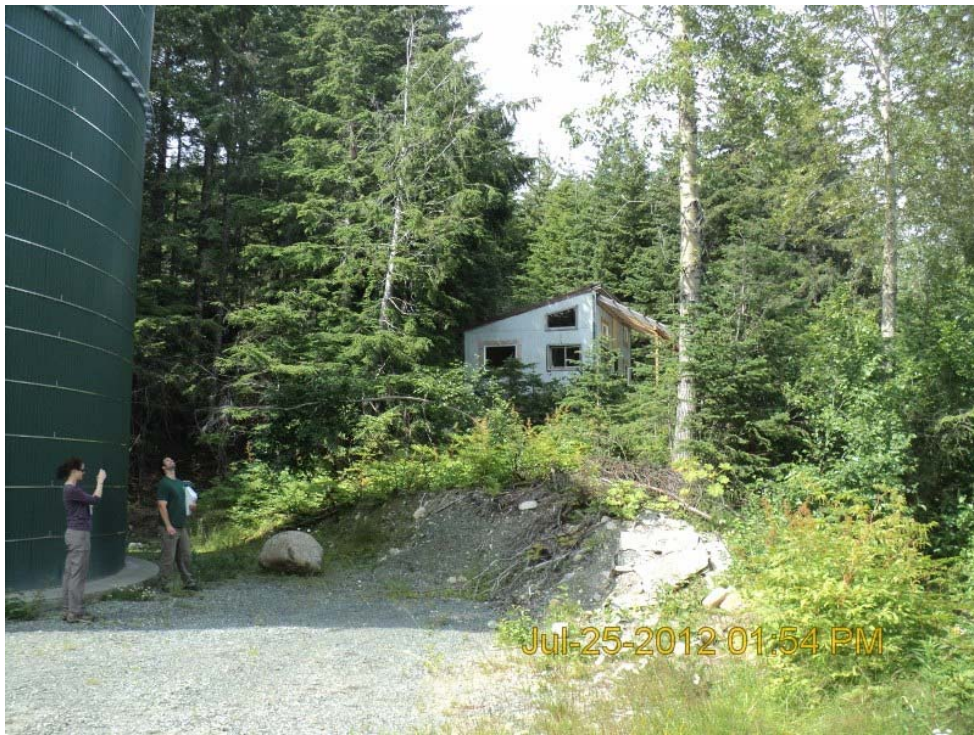
PMP 1.9 (Young Road Site) –Water Tank and Adjacent Soil Berm with Remaining Soil Contamination
