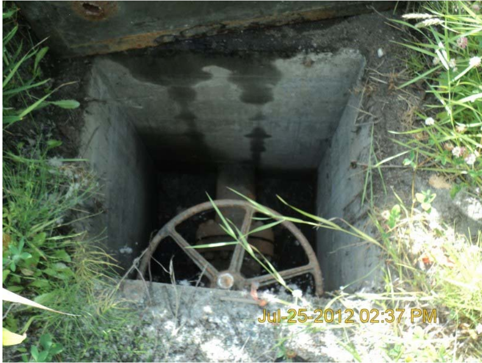
PMP 25.5 – View Inside Gate Valve 4
