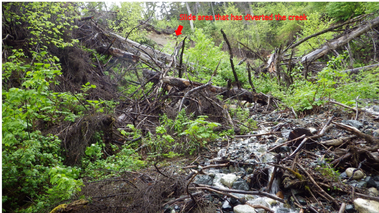
Figure 4. Looking upstream above the highway at stream no. 115-32-10250-2016-3020 headwaters and a landslide. The arrow shows where the slide occurred that diverted the creek.
