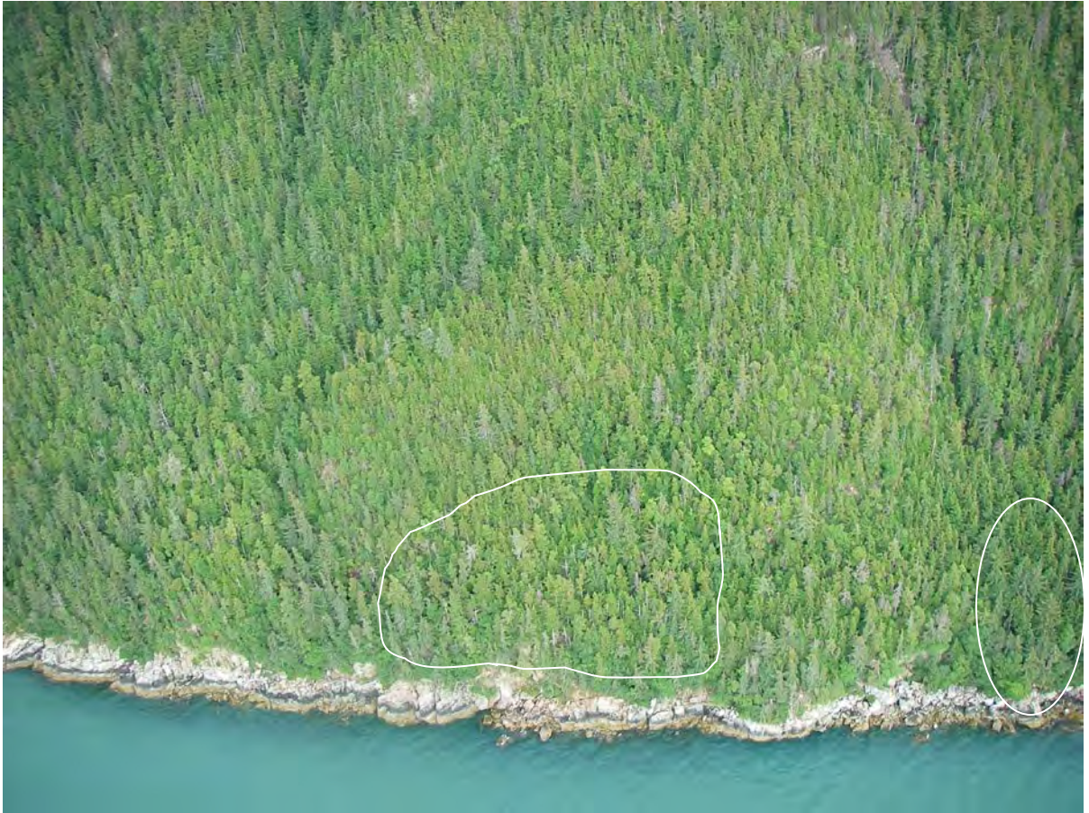
RF39 & RF40. View east/upslope at rockfall hazards RF39 (right) and RF40 (left).
