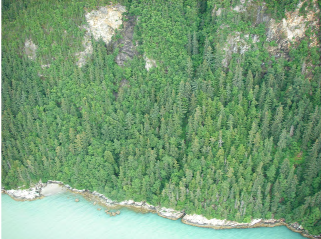
RF52. View east/upslope at rockfall hazard.
