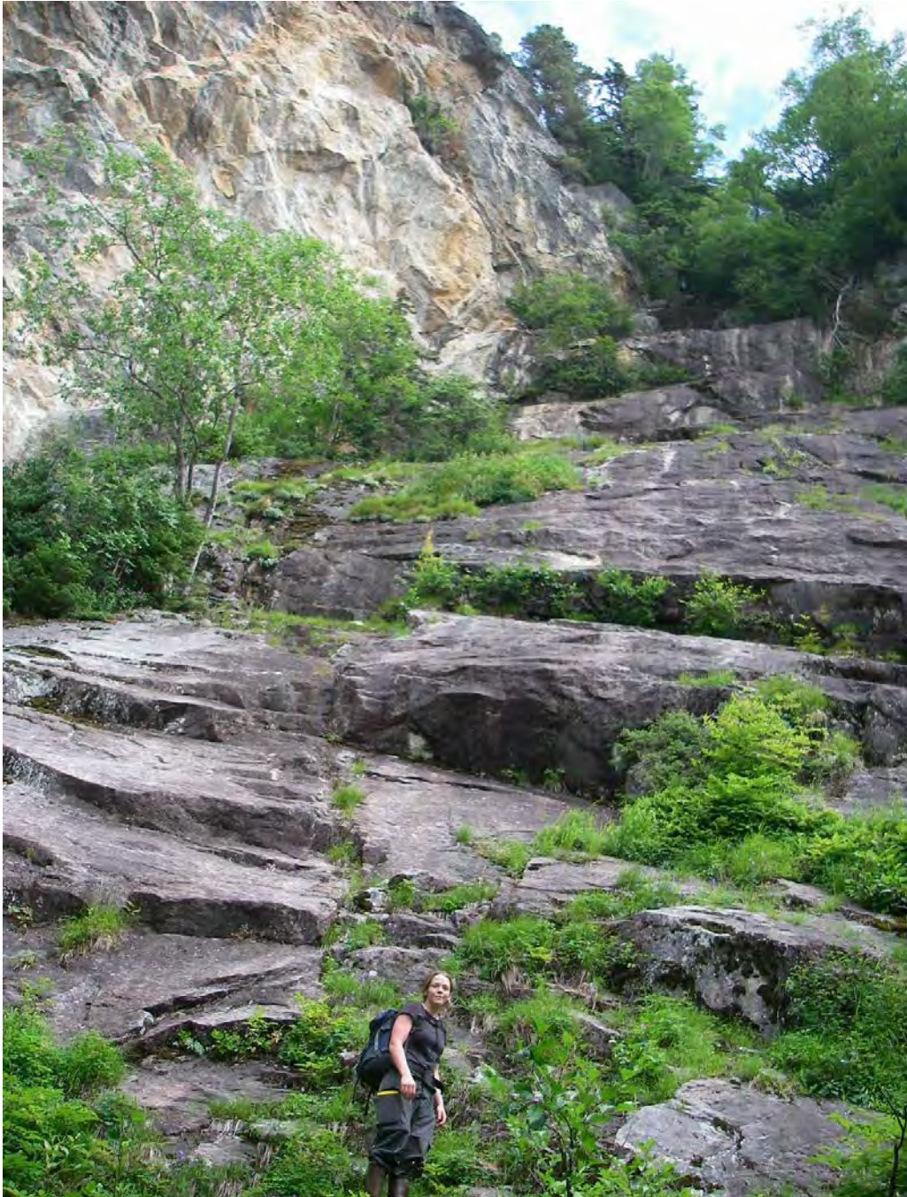
RF52. View east/upslope at source for rockfall hazard. Slope-parallel joints promote planar failure.
