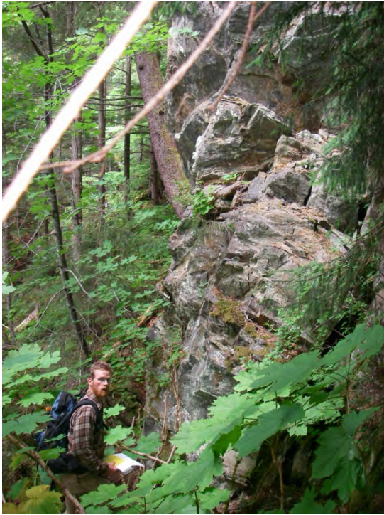
RF46. View north/up alignment at rockfall hazard cliffs.
