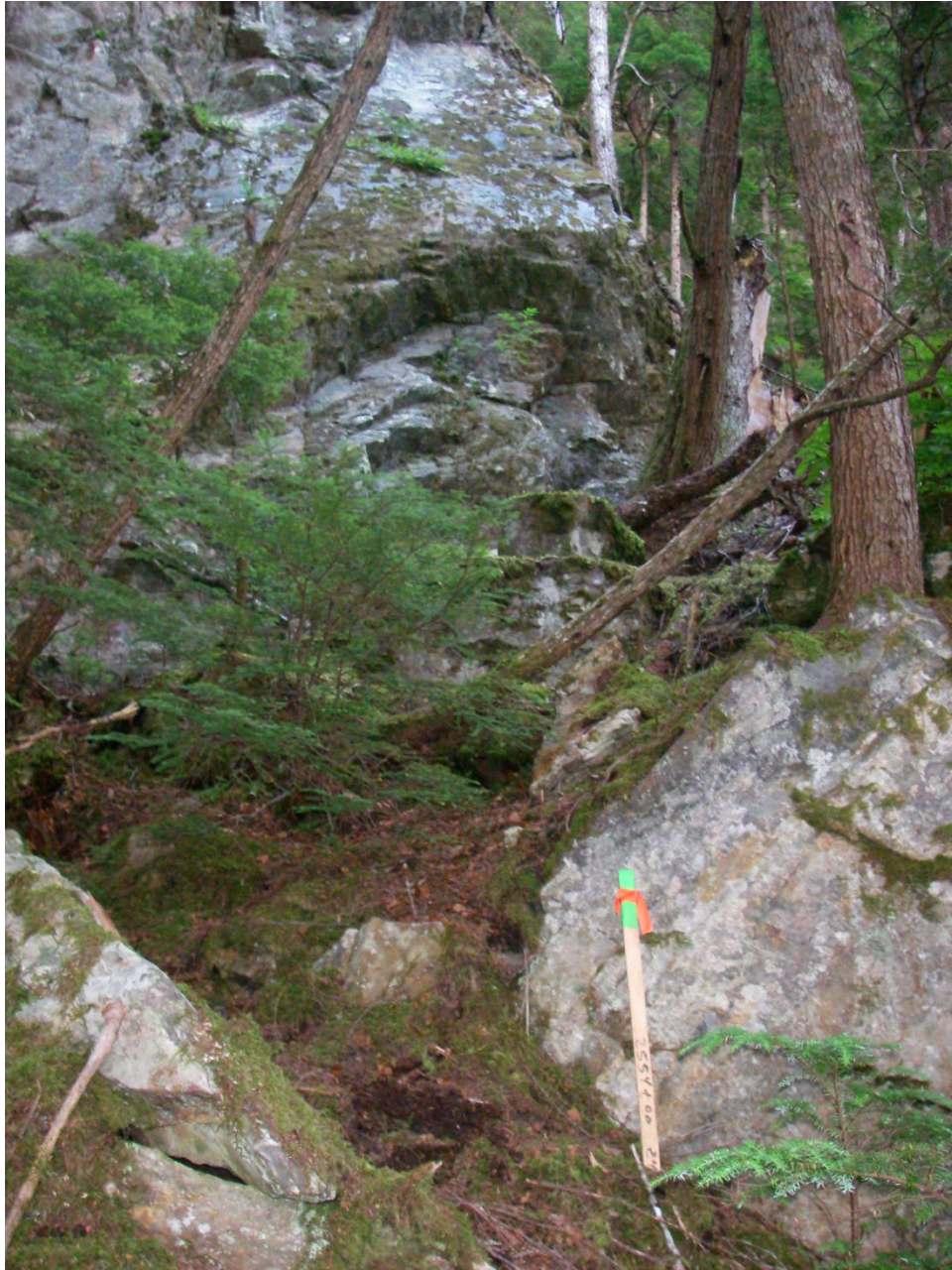
HR05. View east/upslope at hazard rock. Survey lath represents previous IRP 2006 alignment.
