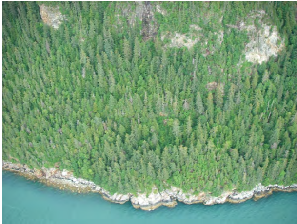
RF42. View east/upslope at rockfall hazard.
