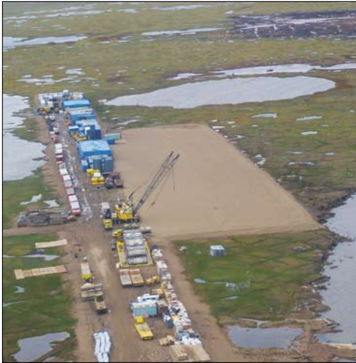
180,000-square-foot pad made of beach sand before treatment.
