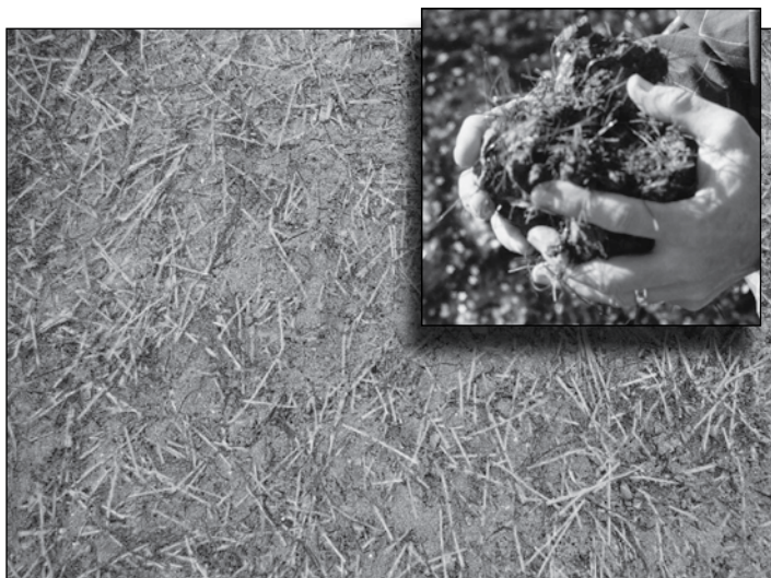
Close-up of blended geo fibers before final application of synthetic fluid and compaction. (continued on next page)
