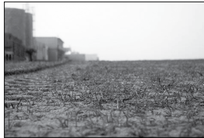
Pad surface after final synthetic fluid application.
