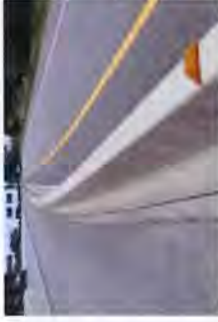
An F-Shaped barrier looks like this.
