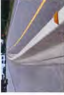
An F-Shaped barrier looks like this.
